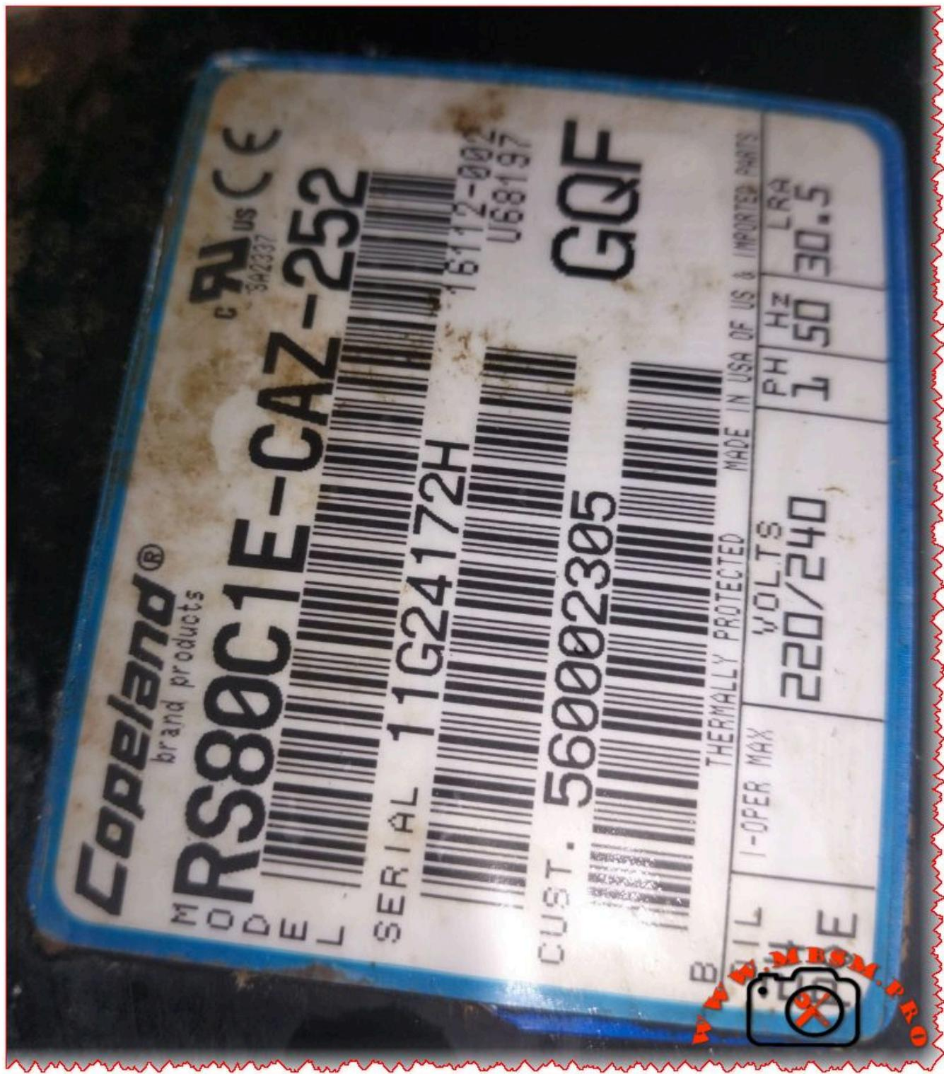
The Copeland RS80C1E-CAZ-252 represents a specialized hermetic reciprocating compressor engineered for low-temperature refrigeration applications where reliability meets efficiency. This single-phase unit operates on R134a refrigerant and delivers consistent performance in demanding freezing environments ranging from -30°C to -10°C evaporating temperatures.
