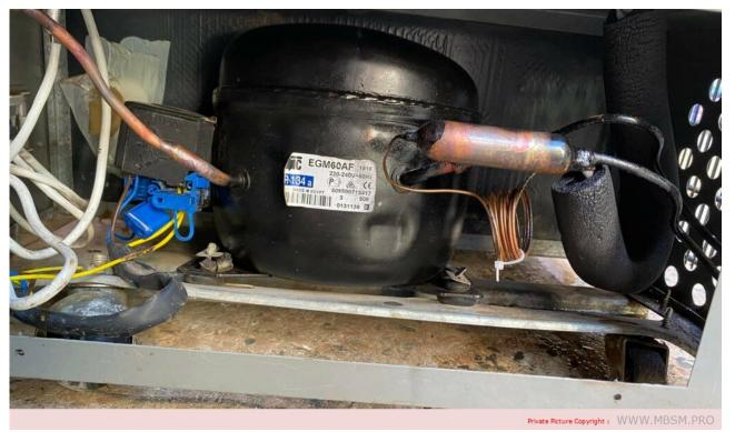
${\tt Mbsm.pro,\ compressor,\ EGM60AF,\ zmc,\ Manufacturing\ Compressor\ Misr\ ,\ 1/6\ hp,\ LBP,\ RSIR\ /\ RSCR}$
