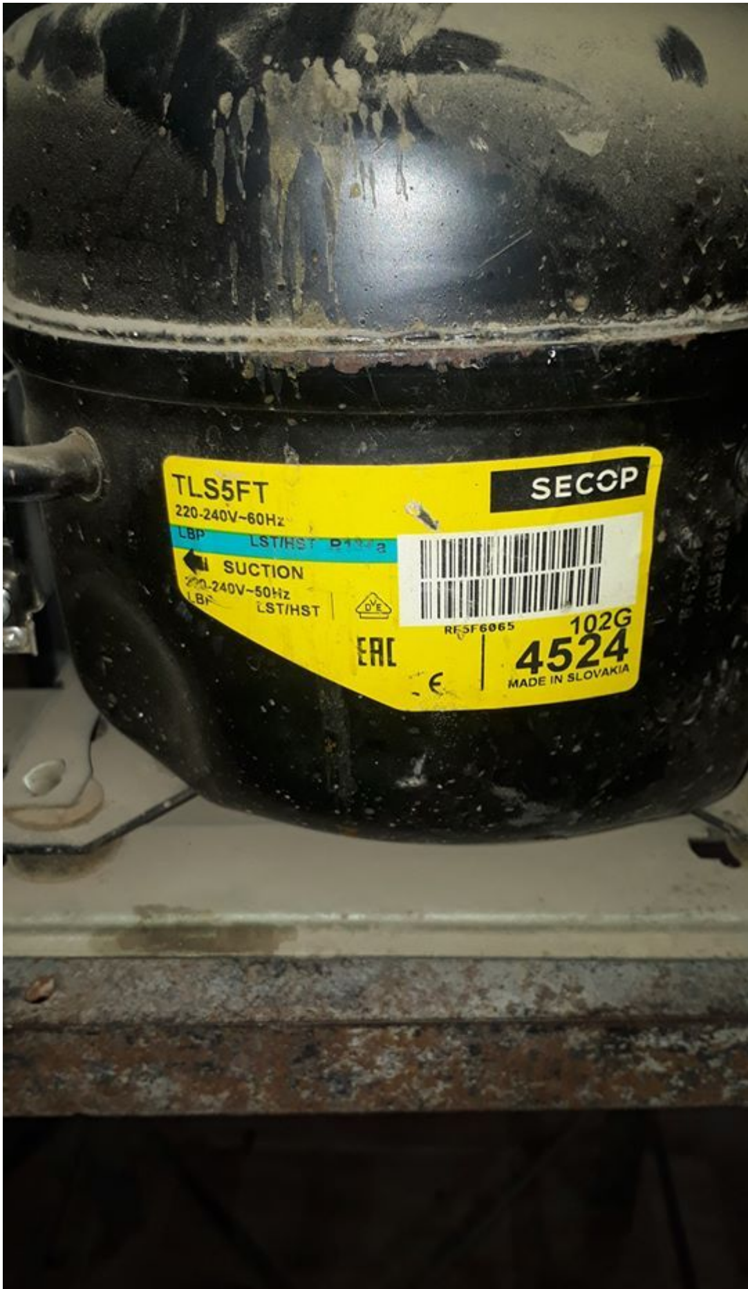
Tropical Compressor ,TLS5FT 102G4524 , SECCP , R134a , 1/6 HP , 134 W , LBP , 220/ 240 V 50Hz
