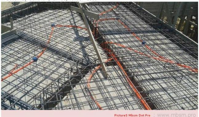
Mbsm.pro,The risk of extending the electric hoses under the reinforcing steel for ceilings
