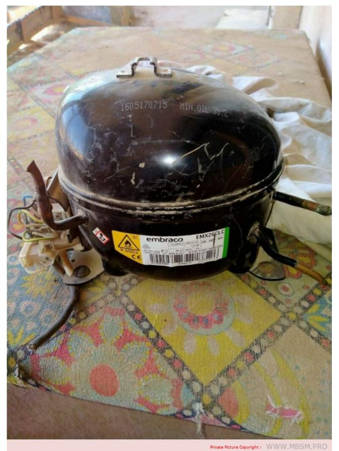
Mbsm.pro, Embraco, Aspera, EMX26CLC, 1/12 hp, single-phase, Compresor, freezing (LBP), 52 crn3, r600a
