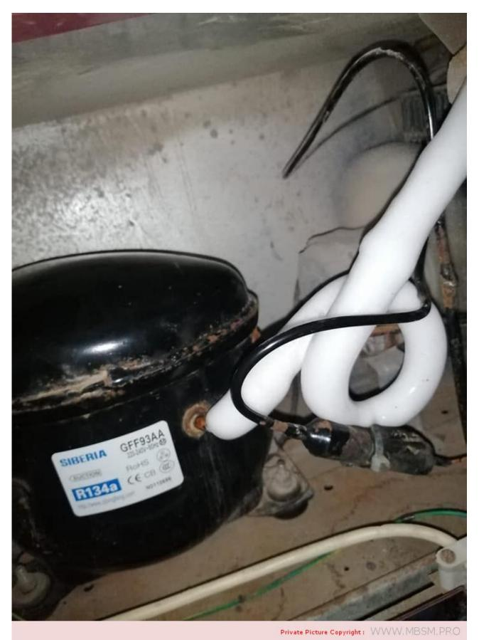
Mbsm.pro, Compressor, Refrigeration Compressor, 270W, GFF93AA, 1/3 HP++, FFI12HBK, TPH1410Y, F Series 200-220V/50Hz, SEBERIA Hermetic Compressor, lbp, hbp
