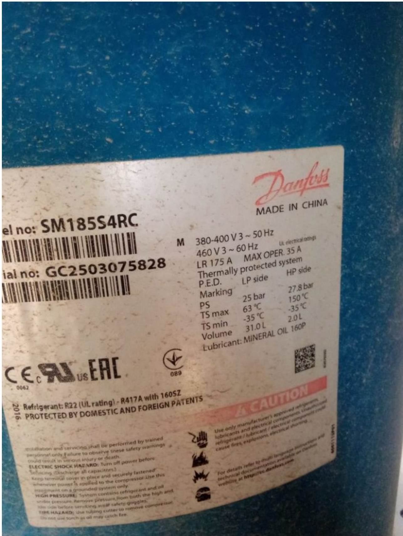
Mbsm.pro, Compressor, SM185, DANFOSS REFRIGERATION, Scroll compressor, SM185S4RC, Danfoss Scroll, 188000 btu/h, R22, 15 hp, 3 ph / 400 v
