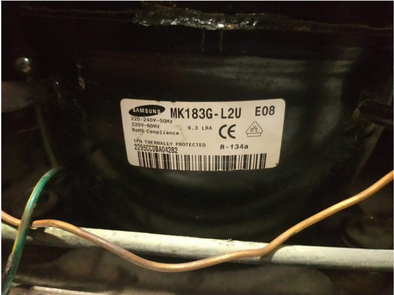
Mbsm.pro, Compressor, Samsung, mk183g-l2u, series MK, 1/3 hp, 236 w, Lbp, 203 KCL, 806 BTU, r134a, 3.8 cc, 220-240V ~ 50Hz, Low Back Pressure, compressor static without fan, PTC-RSCR (Optional RSIR)
