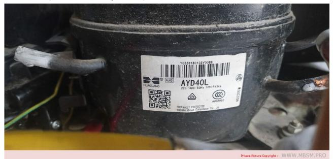
Mbsm.pro, Huaguang, ayd40l, R134A, 220V/50Hz, 1/8HP, 108W, refrigerator, compressor, Wanbao Group Compressor
