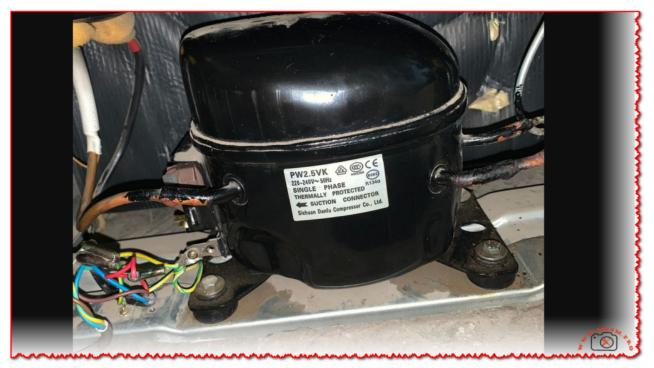
Mbsm.pro, Pw2.5vk, 1/12 hp, Refrigeration, Compressor, R134a,  $220\sim240v$  Ac 50hz, Mbp/lbp, Sichuan Danfu Compressor
