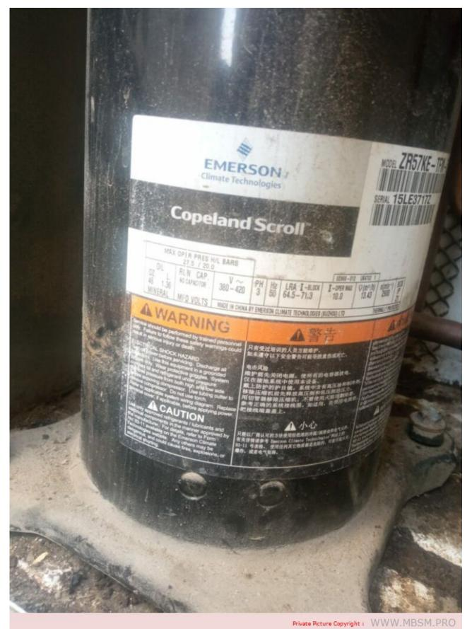
Mbsm.pro, compressor, ZR57KE-TFD, 4.8 hp, 13.900 w, 47500 btu, r22, emerson, copeland, scroll, ZR Series, 380-420□/50H2, 3 Ph
