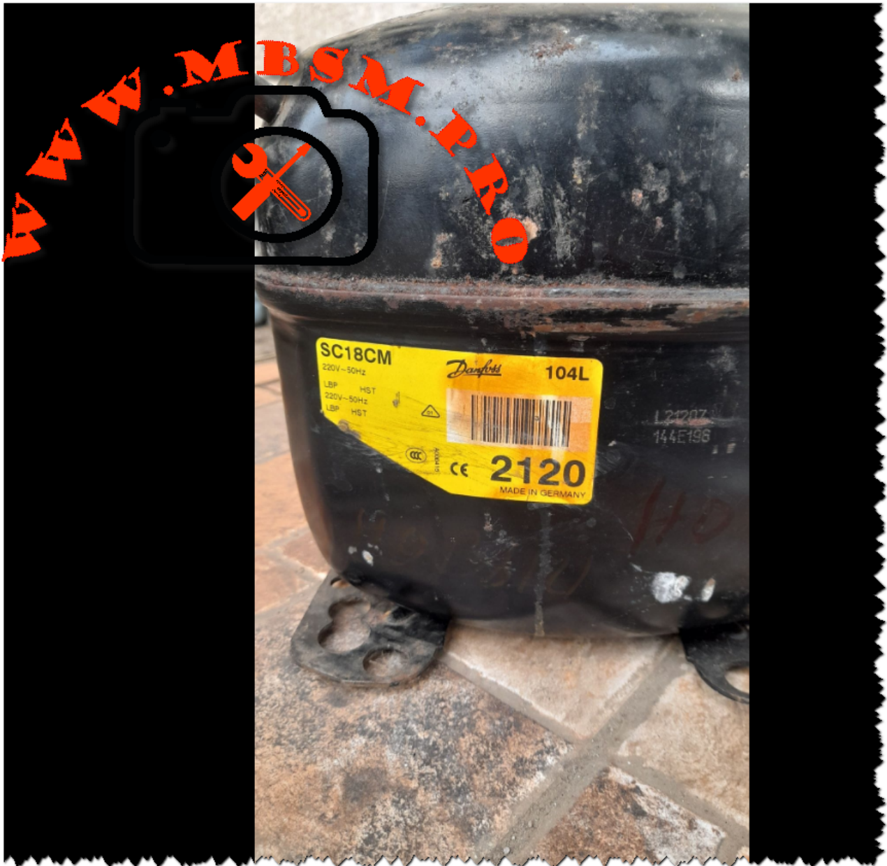
Mbsm.pro, 104L2120, DANFOSS, REFRIGERATION, Reciprocating, compressor, SC18CM, 3/4 hp, lbp, r22, 220v/50hz/1ph
