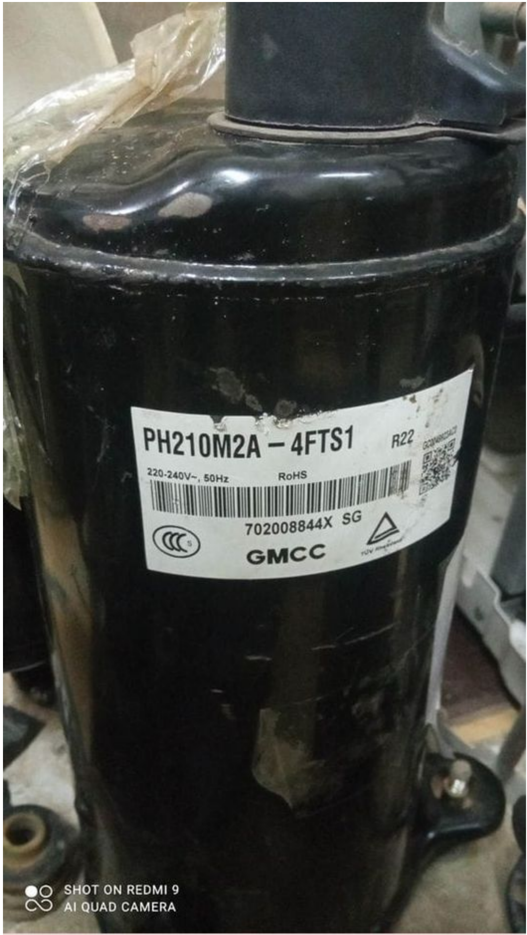
Mbsm.pro, PH210M2A-4FTS1, rotary compressor, GMCC, R22, 1.5 HP, 2.5 A.
