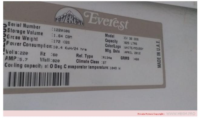
Mbsm.info, upright, double door, cooler, ev32dds, visi cooler, makeeverest, captive, consumption, EV 32 DDS, 825 L, Compressor, 3/8 Hp++, R134A, 460 G, 0.9/1.2 bar, Filtre 30Gr, Capillary, 0.42, 180 psi
