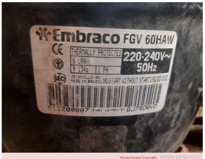
Mbsm.pro, Compressor, FGV60HAW, EMBRACO, 1/5 hp, r134a,
