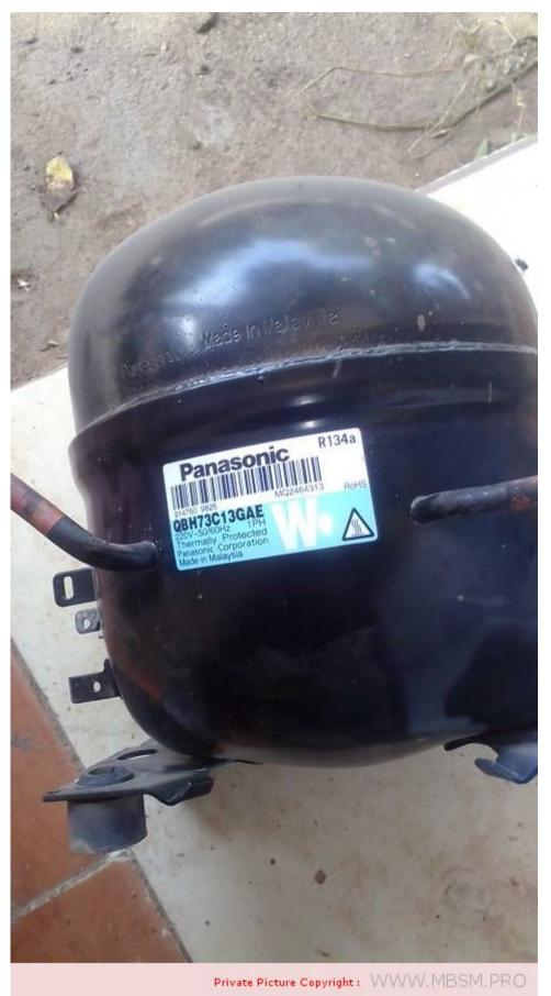
Mbsm.pro, Compressor, QBH73C13GAE, 1/4 hp, RSIR, Reciprocating Compressors, Fixed Speed, Q Series, R134a, LBP
