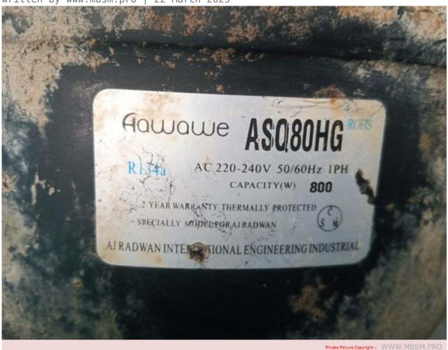
Mbsm.pro, Compressor, Huaguang, asq $80\,\mathrm{hg}$ , Q series,  $800\,\mathrm{w}$ , Hbp, r134a,  $1/4\,\mathrm{hp}$ , cooling Aplication
