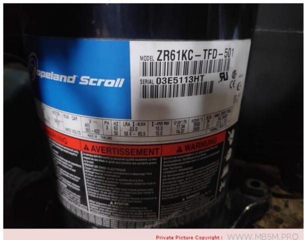
Mbsm.pro, COMPRESSOR, ZR61KC-TFD-522, SCROLL, R22, 3 PHASE, COPELAND, chiller, 14570 w, 49700 btu, 5 Hp
