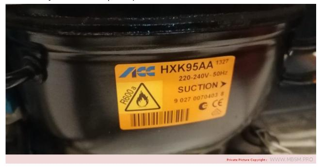
Mbsm.pro, Compressor, HXK95AA, Secop, Danfoss, KAPPA, LBP, R600a, 220-240V 50Hz, 1/6 hp, 129 w
