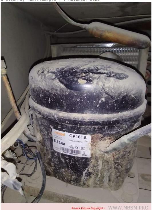
Mbsm.pro, Cubigel, GP16TB, hermetic, compressor, 3/8 hp++, 1/2 hp-, HBP, R134a,
