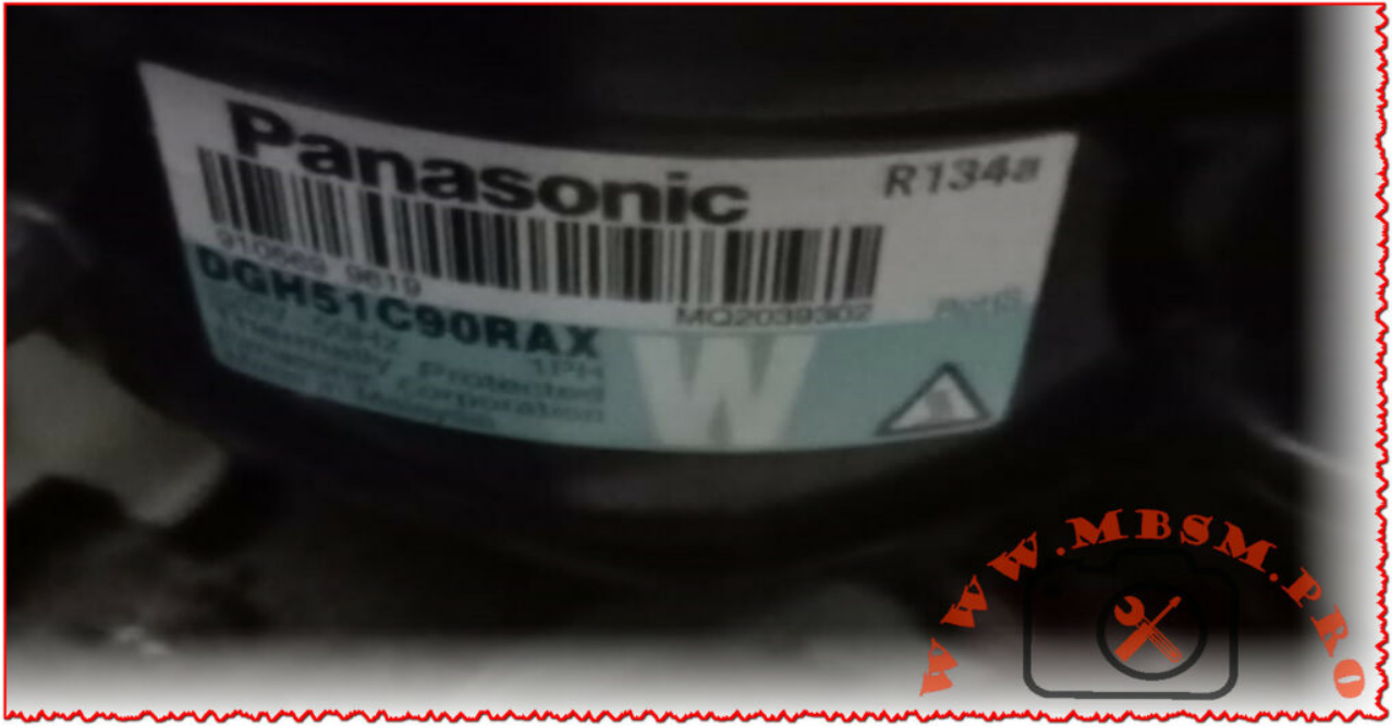
Mbsm.pro, Compressor, dgh51c90rax, 154 w, 525 btu, 132 kcal, 5.1 cm 3 , 1/6 hp, 1bp, Panasonic Compressor
