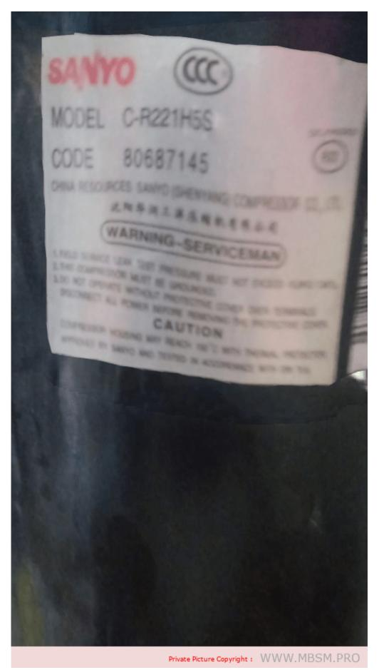
Mbsm.pro, compressor, Sanyo, Rotary, Split system air conditioner, Compressors, C-R221H5S, S6231526791, 24000 btu, R22, 3 hp, 2 ton
