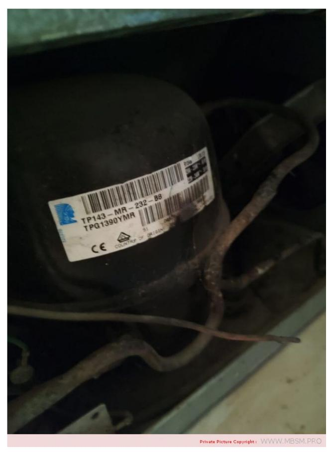
Mbsm.pro, Compressor, Tecumseh, TPG1390YMR, 805 btu/h, 236w, 1/3hp, LBP, Low Back Pressure, R134a,  $208-230V \sim 60Hz$ ,  $220-240V \sim 50Hz$ , Reciprocating Compressor, TP143-MR-232-B8
