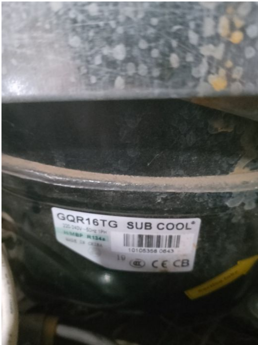
GQR16TG, light, commercial, refrigeration, compressor ,1 / 2+ HP, 220V/50Hz, CSIR, capacitor:80UF, R134A
