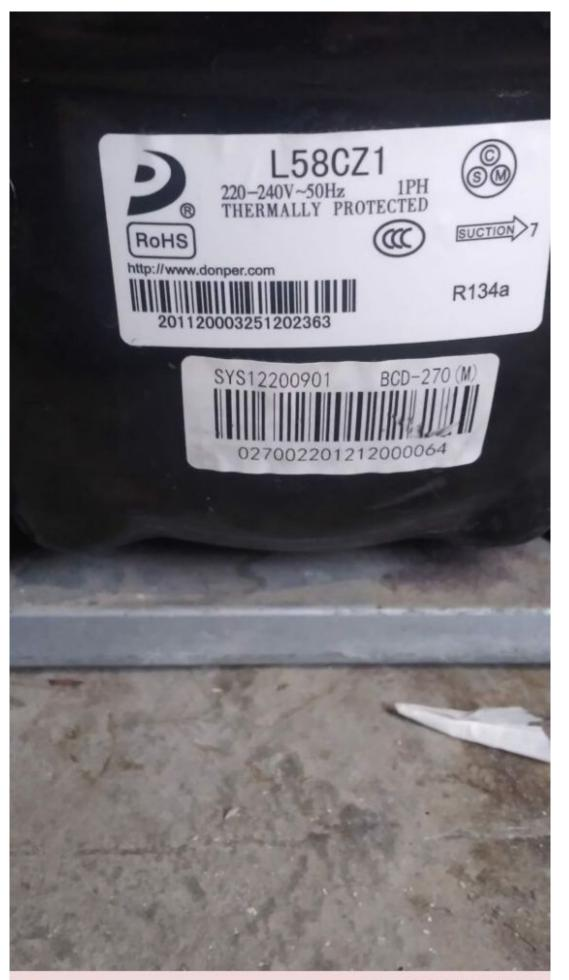
Donper, New, L58CZ1, 220V-240V, 50Hz, R134A ,Refrigerator, Compressor, 1/6++HP, 1/5 hp-, power 116 w, input 145 w
