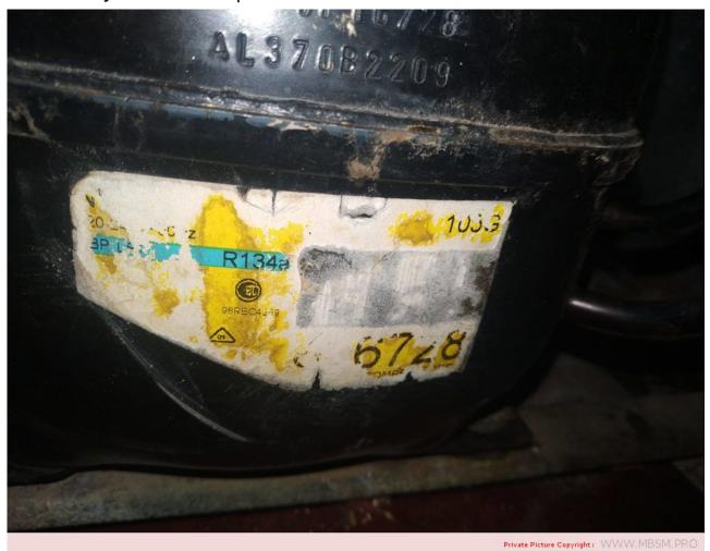
Mbsm.pro, Compressor, 105g 6728, NL7FT, 1/4hp, 105g6728, Danfoss, R134A, 220-240V
