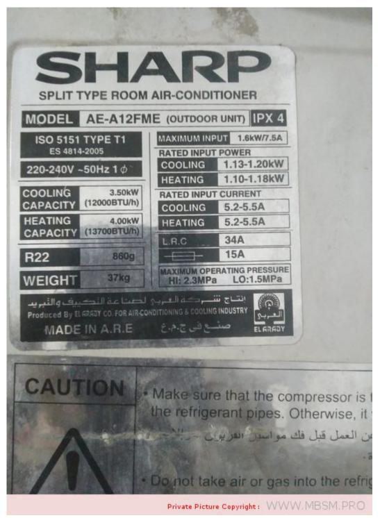
Mbsm.pro, Air conditioner, Sharp, AE-a12fme, 12000 btu, r22, 860 g, 1.5 hp, 1 ton, cooling, heating, T1, PH 1
