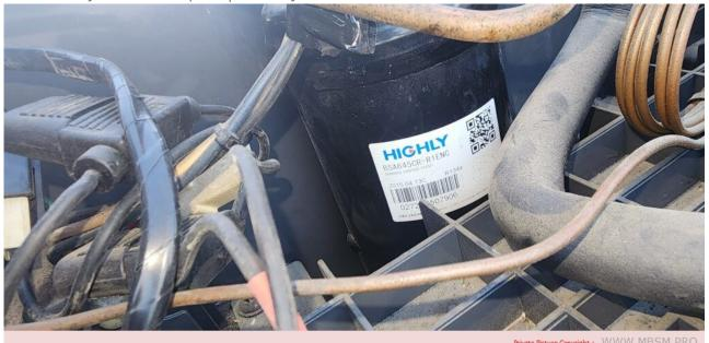
Mbsm.pro, Compressor, HIGHLY, BSA645CR-R1EN, GBSA645CR, 840w, r134a, 1.12hp, Constant-Speed, [1ph] 100/100-110V 50/60Hz
