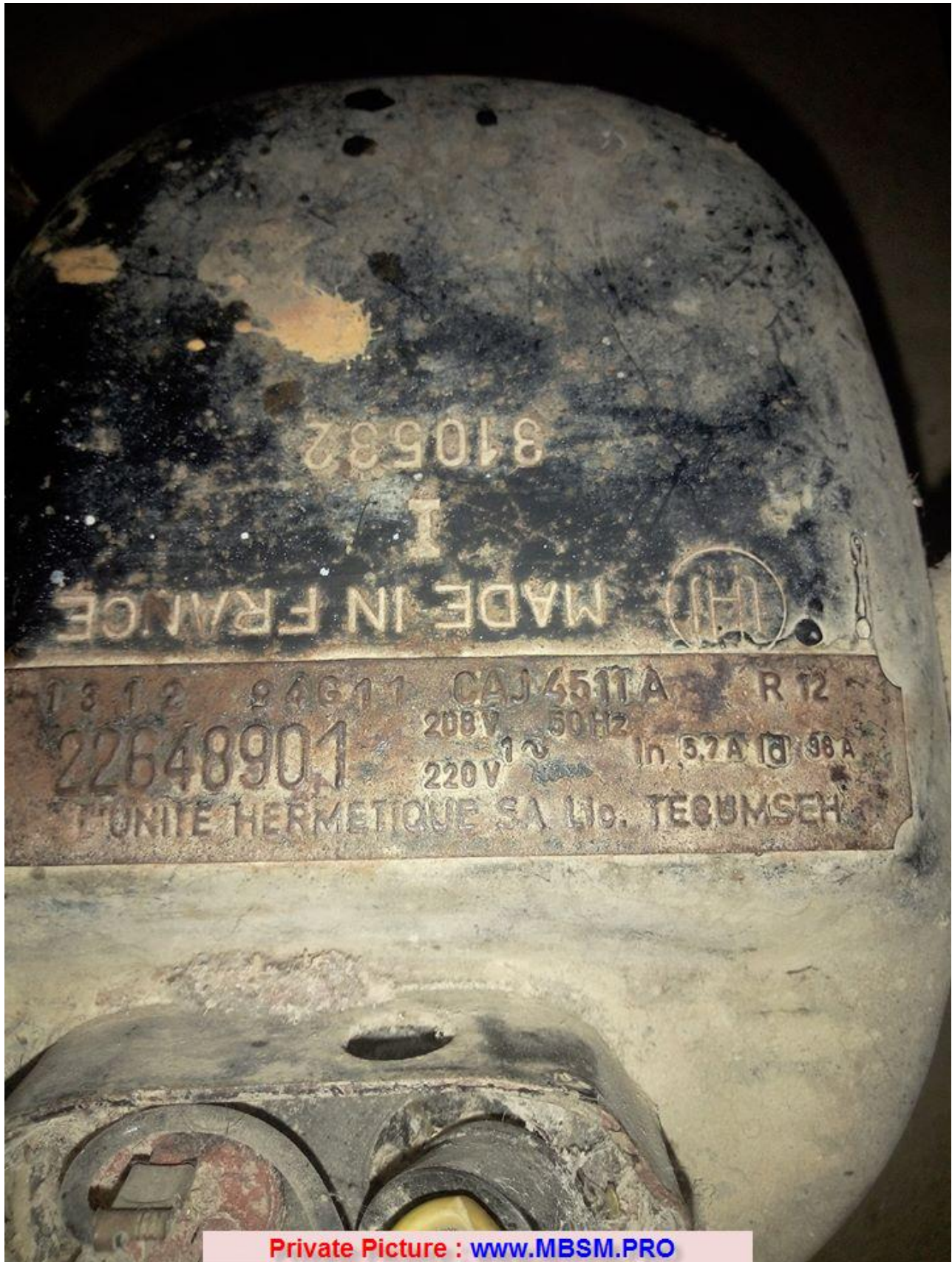
Tecumseh , CAJ4511A ,Compressor , 1 HP, 208-230V, 1 PHASE, R12, Hermetic ,Reciprocating Compressor Replacement
