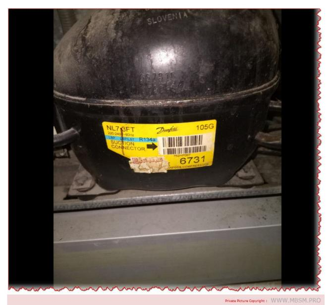
the 105G6731 is a model number for a tropical compressor manufactured by Secop, which is part of Danfoss. Here are the key specifications and details related to this compressor:
