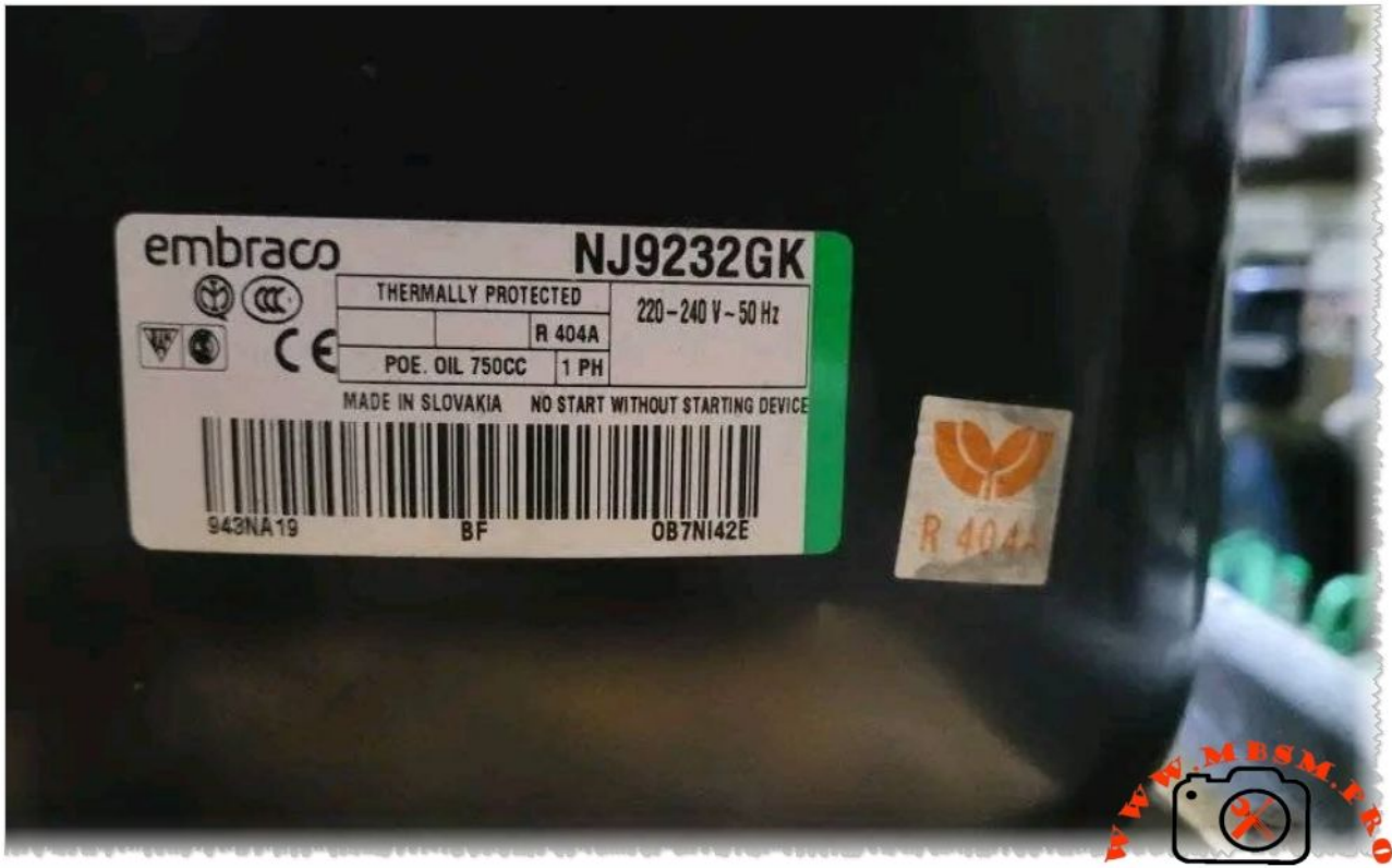
Mbsm.pro, Compressor, NJ9232GK, embraco, 1.1/4 hp, r404, Mhbp
