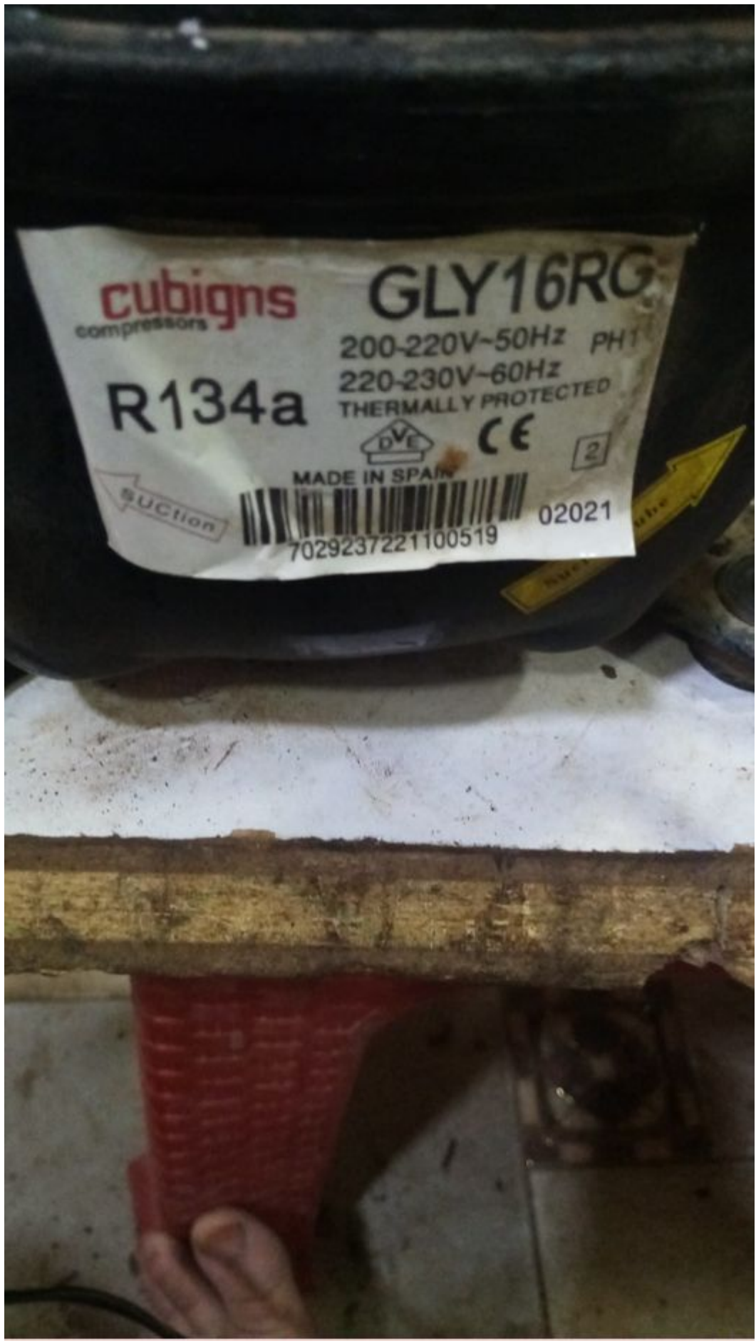
Commercial refrigerator, compressors, GLY16RG, 3/8 hp++, R134a, HMBP, 1492W,
