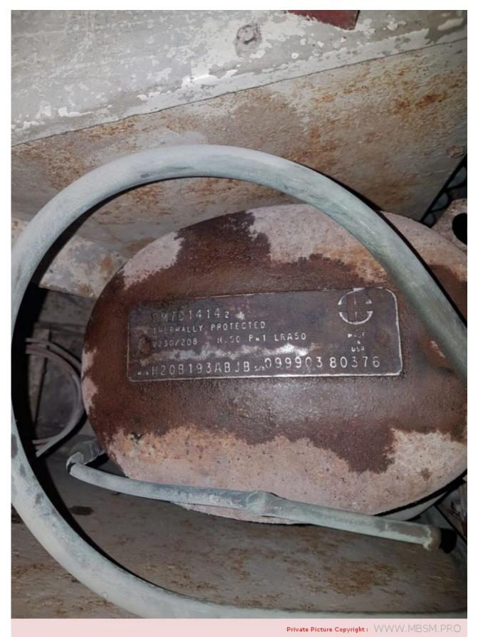
Mbsm.pro, Compressor, H20b193ABJB, bristol compressor, High Temperature, r410a, Third generation, Basic model, Benchmark, 19000 btu/h, psc, 220-240~/50hz, 1 phase,
