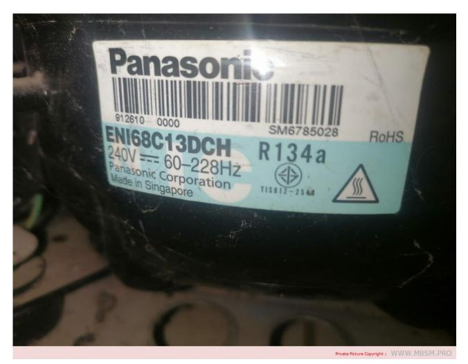
Mbsm.pro, compressor, Panasonic, Lbp, E Series, R134a, ETI57C13DCH, ENI68C13DCH, Reciprocating, Compressors, Variable Speed, inverter, from 63 to 240 w, 240v+-, from 60 to 268 hz, from 25 rps to 72 rps
