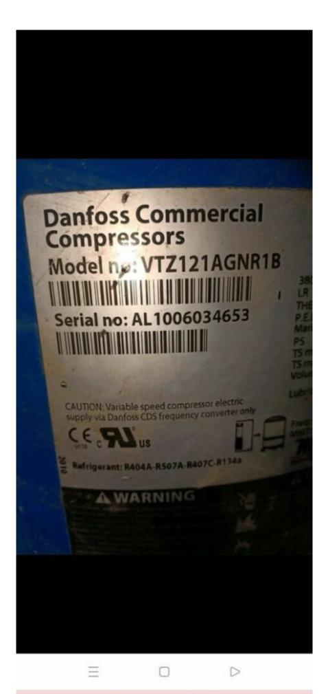
${\tt Mbsm.pro,\ Compressor,\ inverter,\ VTZ121AGNR1B,\ 60000\ btu,\ air\ conditioning}$
