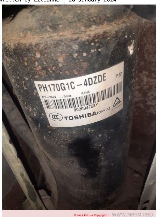
Mbsm.pro, Toshiba, R22, pH170glc-4dzde, Air Conditioner, Compressor, 1 ton, 12000 btu, 1.5 hp
