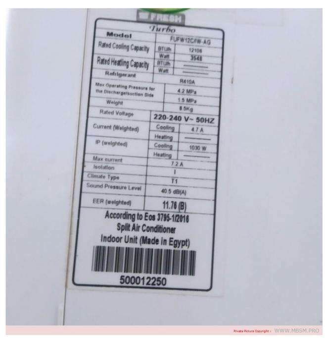
Mbsm.pro, Fufw12caw-ag, air conditioner, Fresh, turbo, Cooling, heating, 12000 Btu, 1.5 hp, 1 ton, r410a, 850 grams
