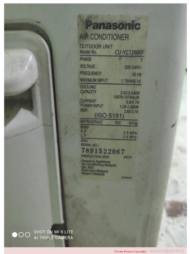
Mbsm.pro, air conditioner, cu-yc12MKF, 12000 btu/h, 1 ton, Cooling only, 8 A, R22, 870 G, 220 v 50 htz, T1, 1/2 copper suction, 1/4 copper discharge
