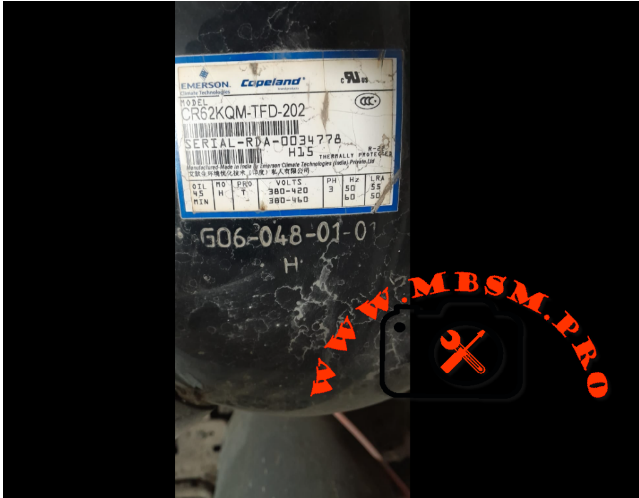
Mbsm.pro , Compressor, CR62KQM-TFD-202, Copeland, Hermetic, 5 hp, 3ph
