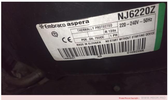
Mbsm.pro, Compressor, embraco, aspera, nj6220z, 3/4 hp++, Hbp, 1hp, 1ph, Cooling, r134a
