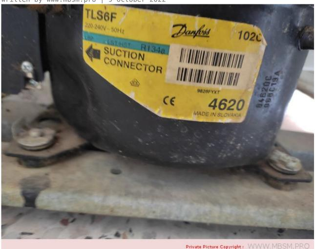
Mbsm.pro, Compressor, TLS6F, Danfoss, 102G4620, Lbp, 125 W, 220 v, 1/6 Hp, 1 phase, R134a
