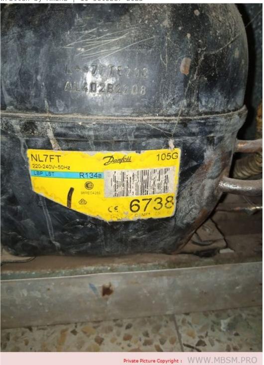
Mbsm.pro, Compressor, 1/5 Hp, NL7FT, SECOP, DANFOSS, 105G6728, 105G6738, Lbp, r134a
