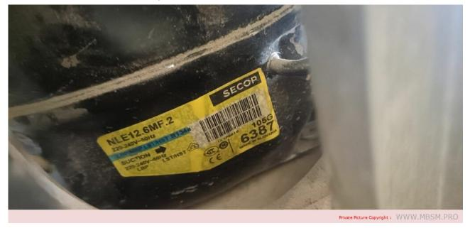
Mbsm.pro, Compressor, NLE12.6MF.2, SECOP, 105G6387, DANFOSS, R134a, 1/2 Hp, lbp
