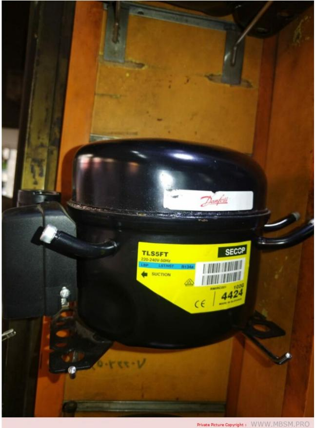
Compressor, TLS4FT, SECOP, 102G4424, 102G 4424, DANFOSS, 1/8 hp++, 98 w, lbp, r134
