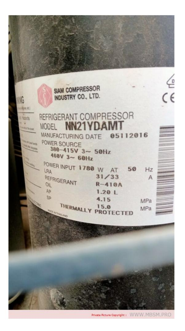
Mbsm.pro, R-410A, Fixed Speed, Rotary, Compressor, Mitsubishi, NN21YDAMT, 1.74 hp, 18000 btu, 3 Ph, 380 v
