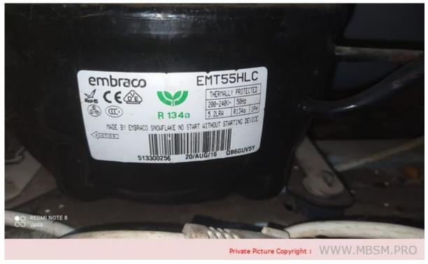
Mbsm.pro, Compressor, Refrigerant, 1/5 hp, R134a, EMT55HLR, 220-240V 50Hz, 1PH, Embraco
