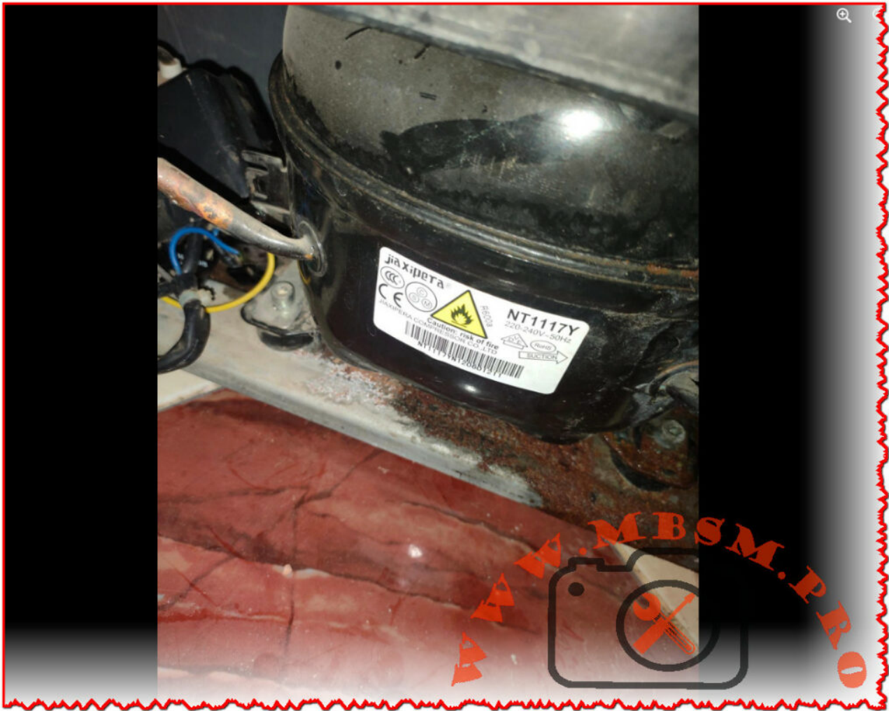
Mbsm.pro, refrigerator, RD-73WS4S, Hisense, 597 L, R600a, 58 g, 230 w, Compressor, Nt1117y, 1/4 hp
