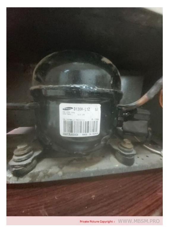
Refrigeration, Compressor, 1/10 HP, R-134A, Samsung, CD130C-L1Z2
