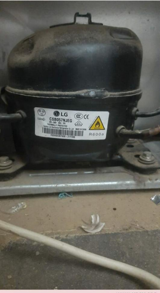
Mbsm.pro, Refrigeration, compressor, 1/10 hp, CSB Series, freezer, 100W, R600a, 5.7cm3, 1PH, Beko, Candy, LG, CSB057NJEG (1/10HP), CSB069NJEG (1/8HP), Lbp, small compressor, Water Purifier Commercial Refrigeration, SMTB-150, 105 L, r600a/25 g, T class, 0.5 A
