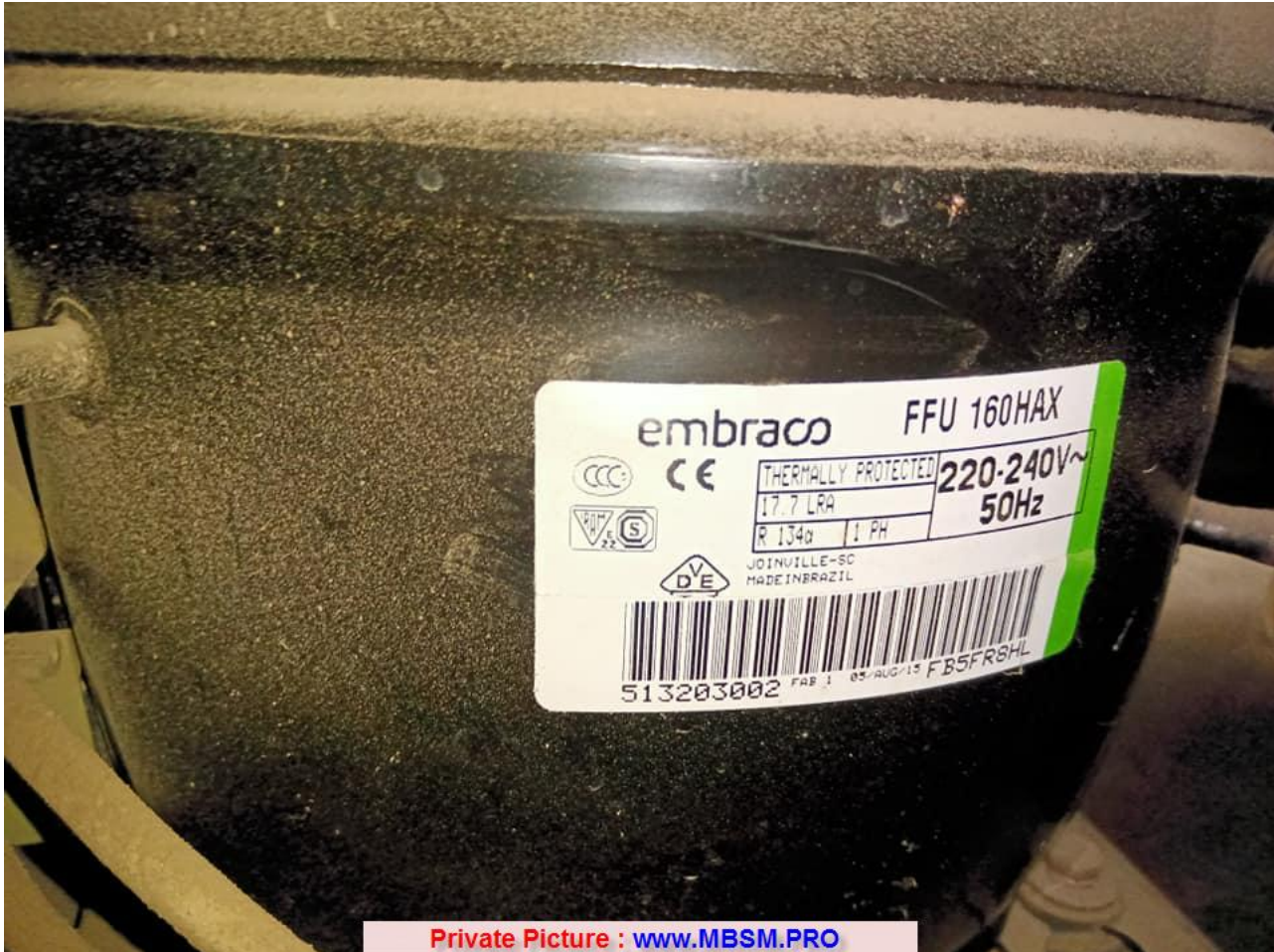
Compresor Embraco, T/M-B FFU160HAX 1/2 HP,1,533 BTU/h,R-134 A ,MBP
