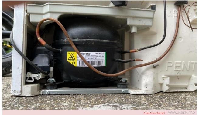
Mbsm.pro, Compressor, TLX4KK, 102h 4446, Compressor Mini Portable, R600A, Truck Car Fridge, 20-to-40 L, Compatible , EMY20CLC, 1/12 hp, Lbp, 54 W at  $23^{\circ}$ C, Capacitor 2,5 $\mu$ F
