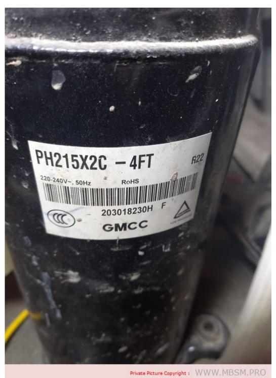
Mbsm.pro, Gmcc Rotary, Compressor, Gmcc A/C , R22, 220-240V/50Hz, 12000BTU, pH215X2C-4FT
