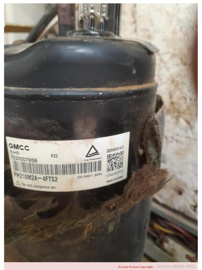
Mbsm.pro, Compressor, Ph310M2A-4FTS2, T3, R22, Toshiba, Gmcc, Rotary Compressor, for Air Conditioner, 1765 w, 19000 btu/h, 50HZ-220/240V
