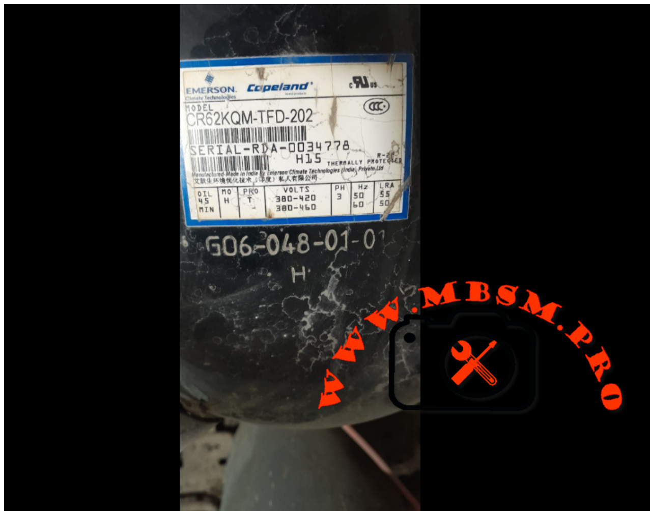
Mbsm.pro , Compressor, CR62KQM-TFD-202, Copeland, Hermetic, 5 hp, 3ph
